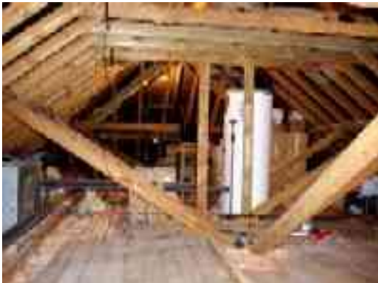
Antenna and Attic installation
